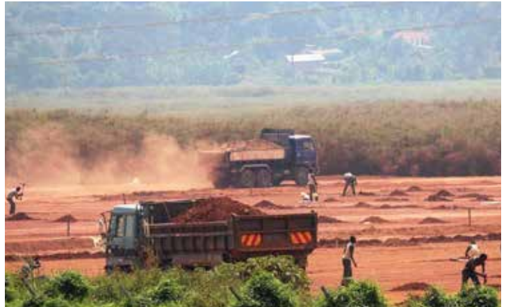
A section of Lutembe wetland being degraded permanent in 2012 to create room for flower growing
